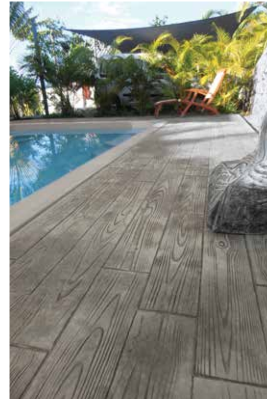
DuraPrint makes it possible to create reliefs, textures and colours on fresh concrete.
